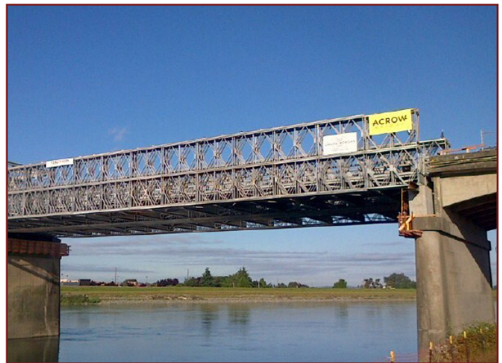
Top: Skagit River I-5 Bridge collapse. Bottom: Completed temporary replacement of the Skagit River I-5 Bridge. Photos courtesy of the Washington State Department of Transportation.
